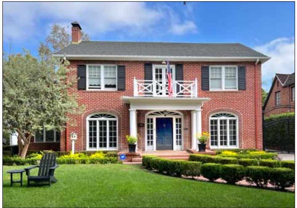
This home at 2445 North Park, built in 1927, is a classic example of Colonial Revival architecture.
