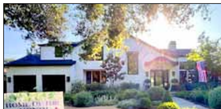
2220 North Heliotrope Drive
